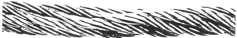
Crushing. Because of loose winding on drum, rope was pulled in between underlying wraps and crushed out of shape.
